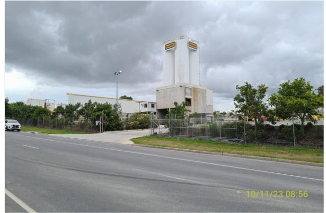
Concrete Crossover Entry
