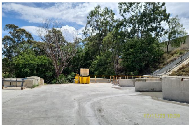
Wash Down Area with Undevelopable Component at rear
