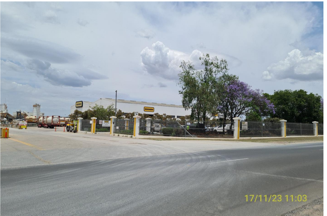
Site View Photo as at Date of Inspection (17 November 2023)
